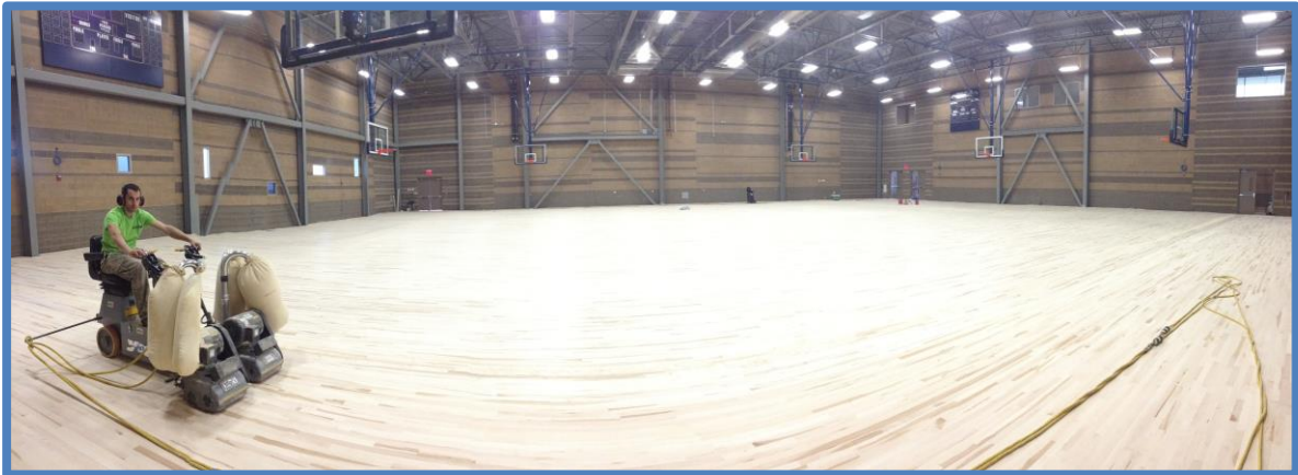
A Horner floor being sanded down
