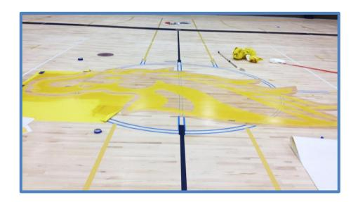
Then, a special tape is laid so that the bulk of the mascot design can be stained with sharp edge lines.
